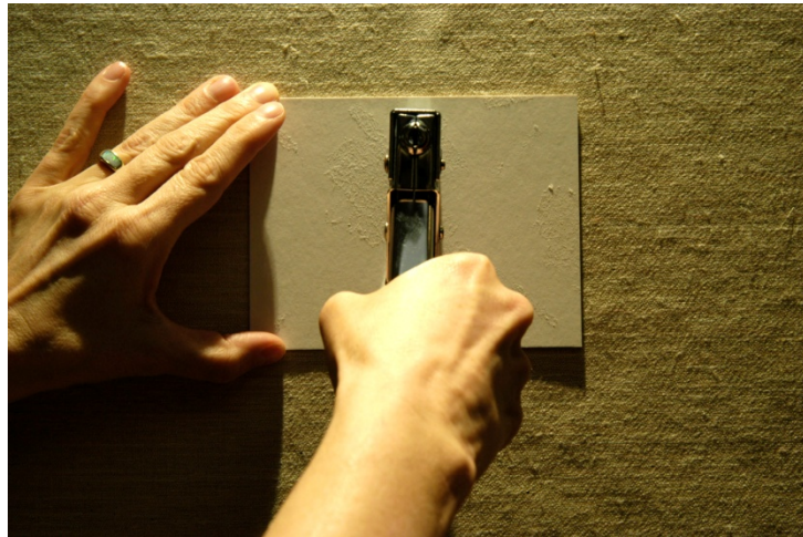
Stapling the mounting plate to the exhibit wall back
