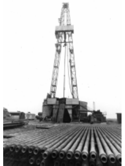
Photo shows a boring operation held in Anju, North Korea.
